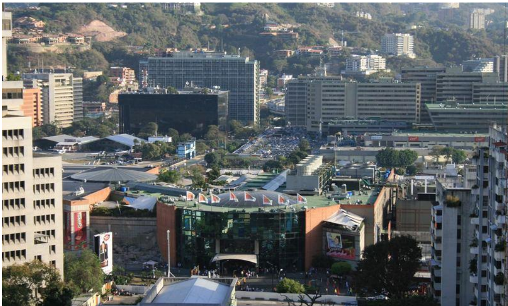
Figura 21 Vista al techo del CCS. (skyscraperlife, 2012)
