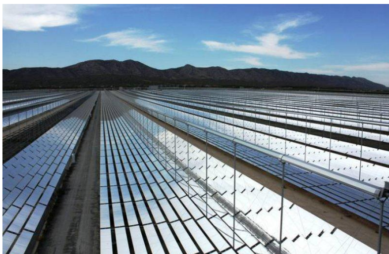
Figure 6. Fresnel power plant in Southern Spain (Puerto Errado 2, source: www.csp-world.com)
