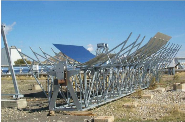
Figure 21. Space frame structure of a Eurotrough collector module (source: Gunther et al., 2011 ).
