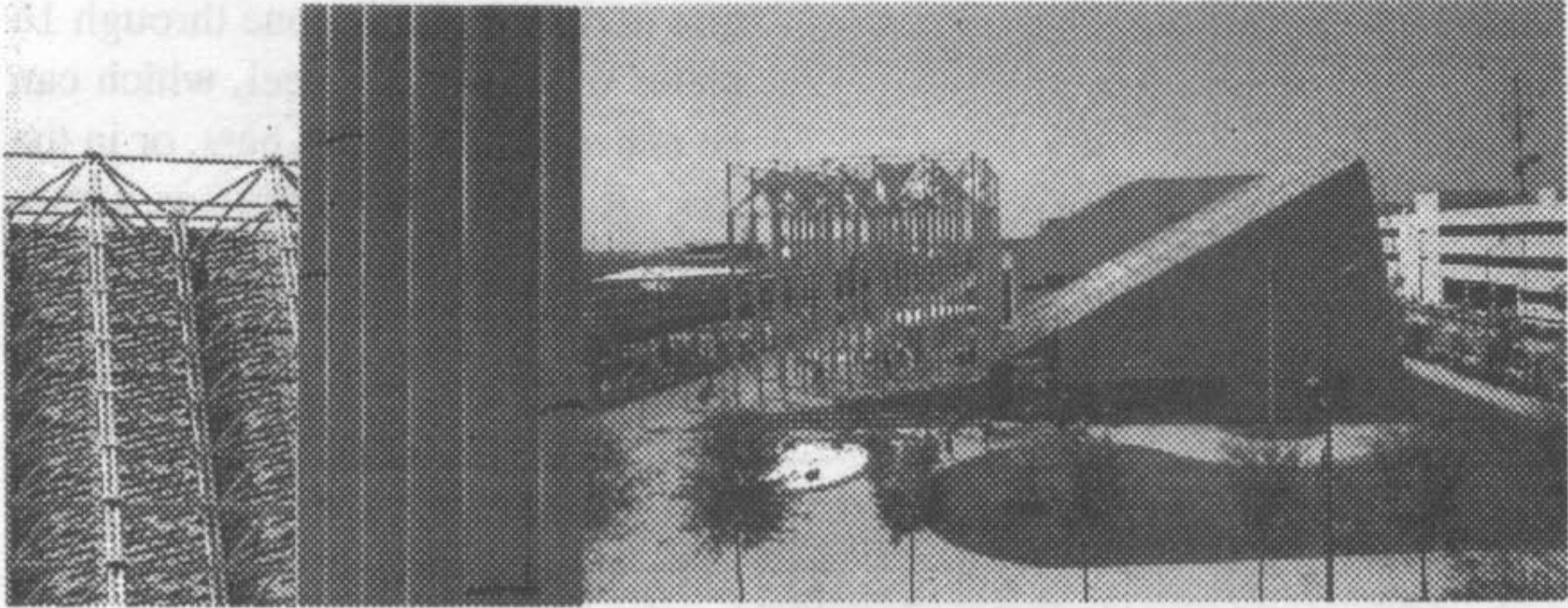
Fig. 9 View of structure
