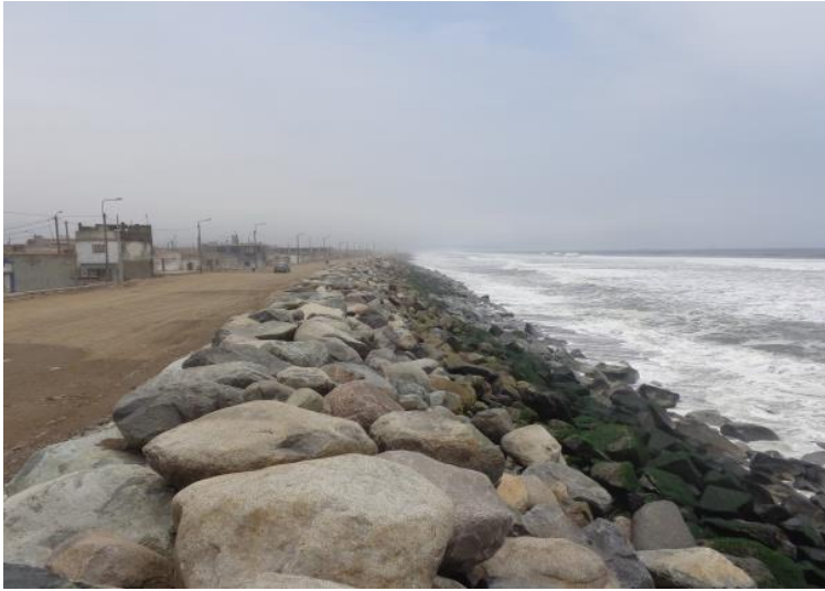
Figure 7. Protection infrastructure with rocks to prevent erosion and destruction of the houses on the beach in Buenos Aires, Trujillo. Photo taken in September 2015 (Photo: F. Benites).
