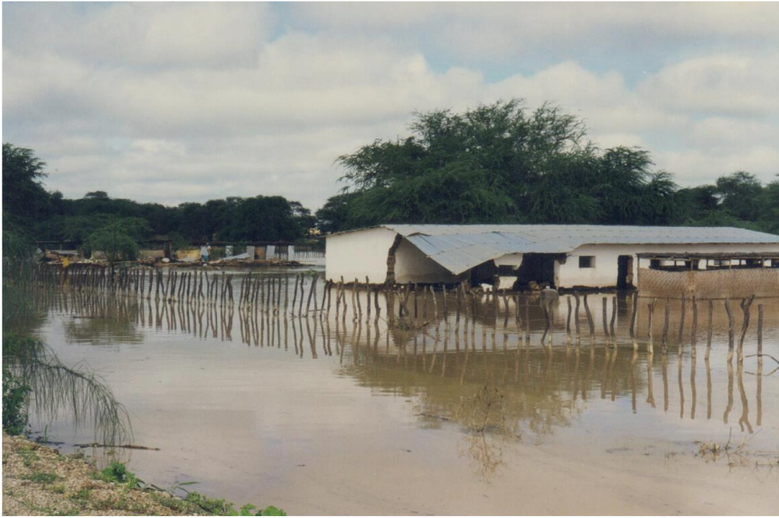
Figure 1. Heavy rain causing landslides and floods in Piura highlands in January of 1998. (Photo: A. Indacochea).
