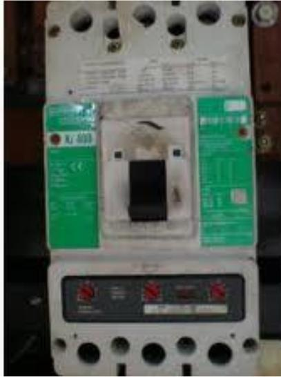
Figura 2.8 Interruptor termo magnético FI Cutler Hammer [21]
